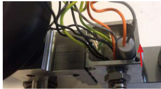
Removing the heating resistance
